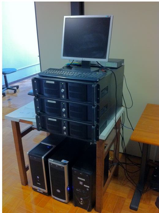
Figure 5.5: Xen testbed physical installation.
